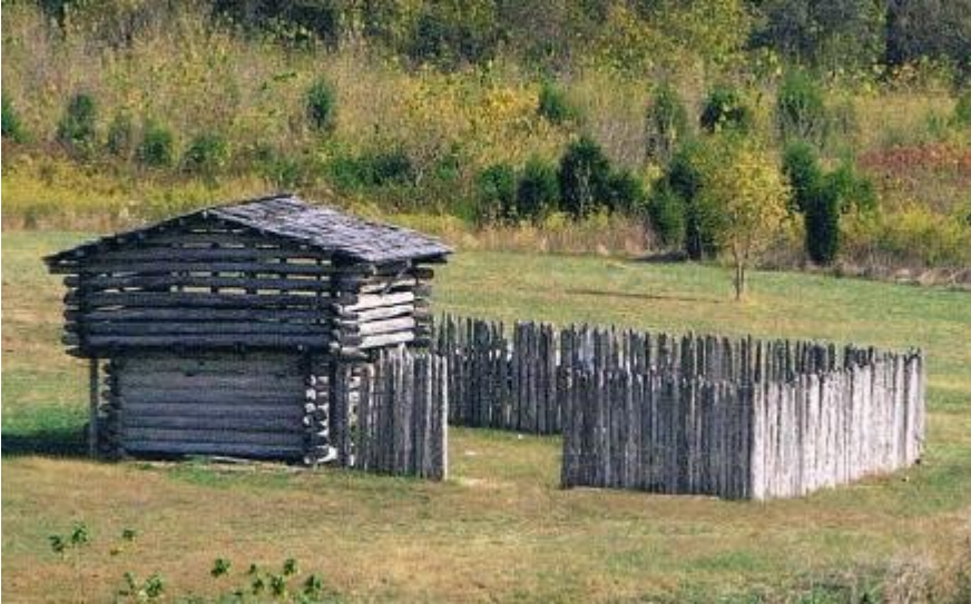
Front view of the reconstructed Tanner Station built in 2003.
