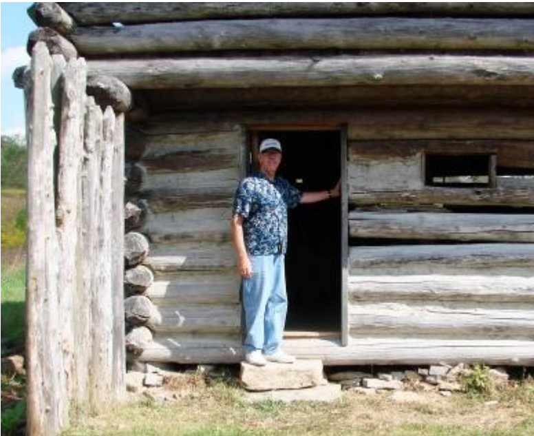
Compatriot Gary Tanner seen here in the doorway of the two-story blockhouse of the reconstructed Tanner Station.
